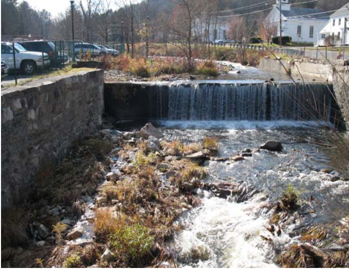
Ballou Dam – Before
