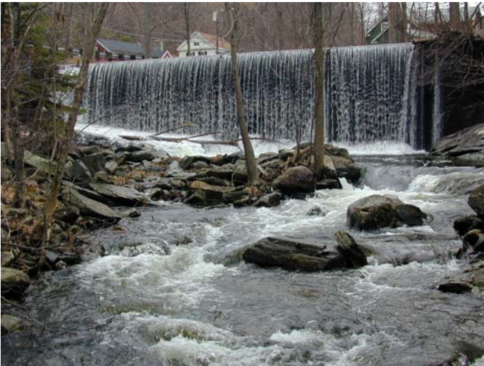
Silk Mill Dam – Before
