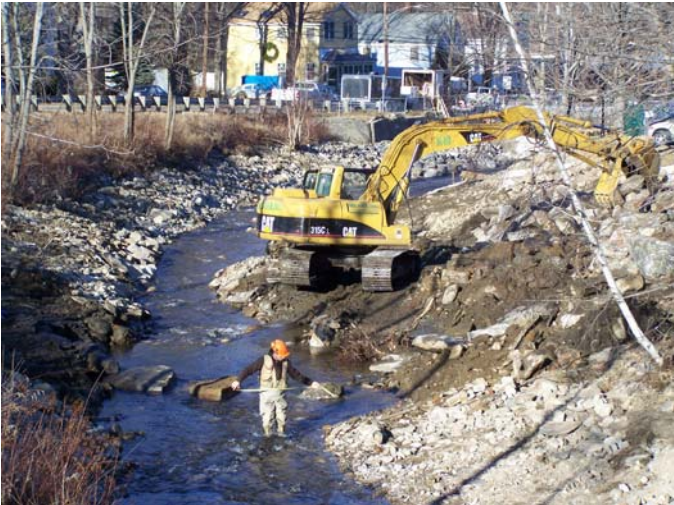
USFWS Staff Installing Step Pool
