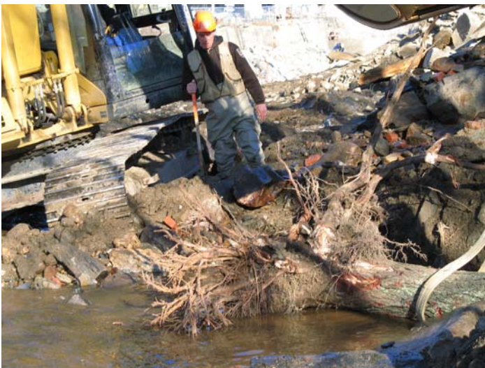
Habitat Structure Installation for Salmon
