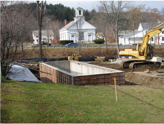
Cistern Installation for Fire Suppression
