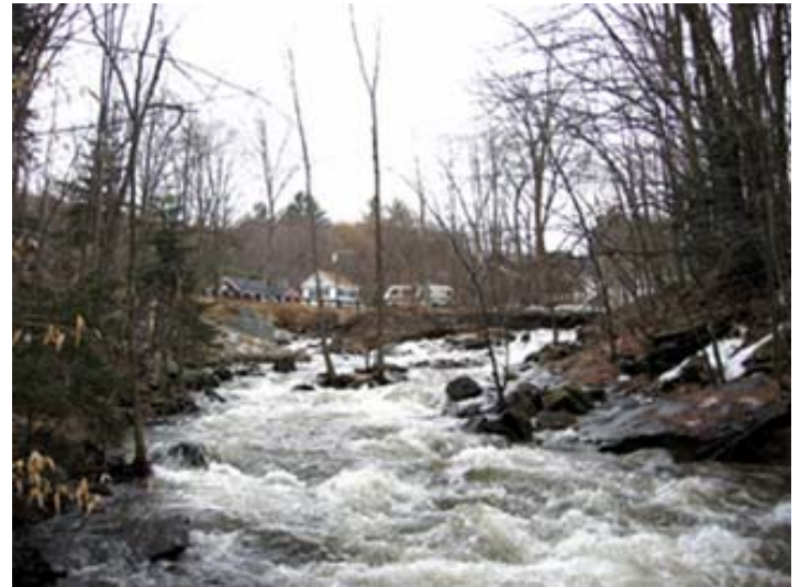
Silk Mill Dam - After
